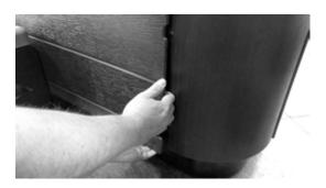
**Step 3:** Electrical Disconnect – be sure to disconnect any lighting or any other electrical wiring that is mounted onto the door before completely removing it.
