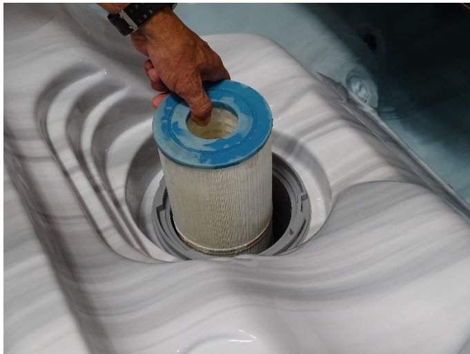
Figure 16. Drop in filter removal
