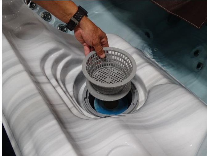
Figure 15. Basket removal
