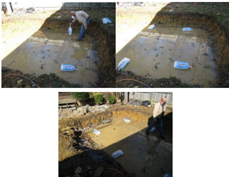
Figure 7. Ice Bag Positioning in Excavation
